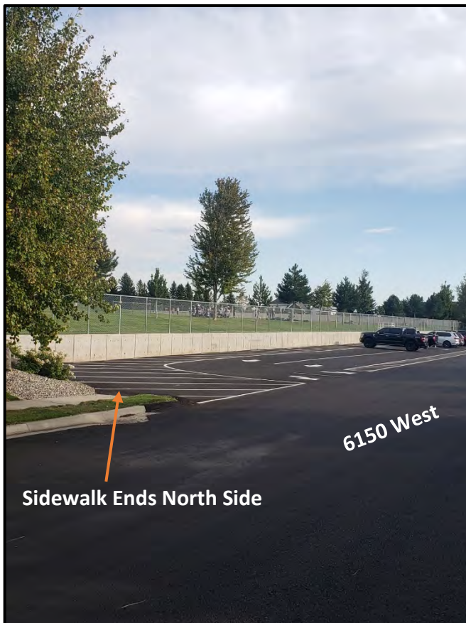
Figure 5 – 6150 West (Back Entrance of School) Facing South, After Highland City's 2021 Pavement/Drop-off Zone Project.
