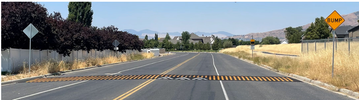
Figure 4: Photo of East Speed Table (Facing West)
