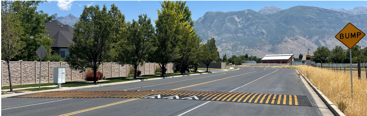
Figure 3: Photo of West Speed Table (Facing East)
